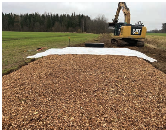
Construction of a woodchip bioreactor
